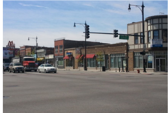
Upgraded traffic signal equipment at Cicero/Irving Park/Milwaukee
