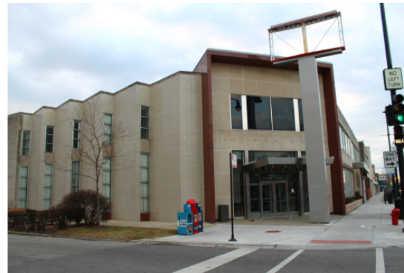
The former Bank of America facility at 4901 West Irving Park Road
