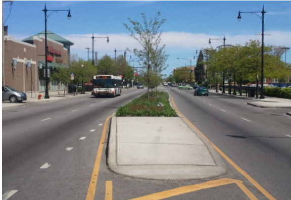
Median planter on Cicero where pedestrians regularly cross east-west unprotected
